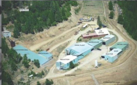
ANTIMONY SMELTER PLANT - THOMPSON FALLS, MONTANA
