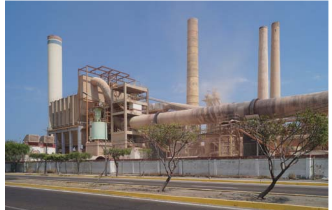
Cement Plant By Rjcastillo
