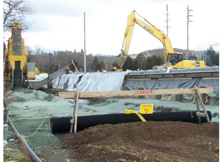
PTW construction at WVDP Reprinted with permission from Alan Rabideau, University of Buffalo, Buffalo, NY.
